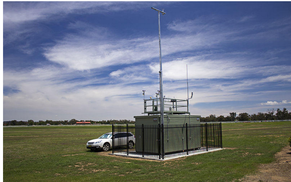
Air monitoring station
