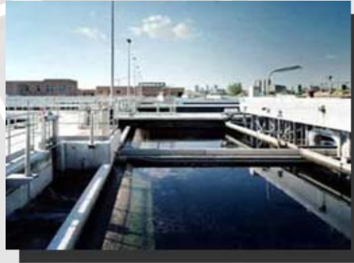
Sewage treatment plants
