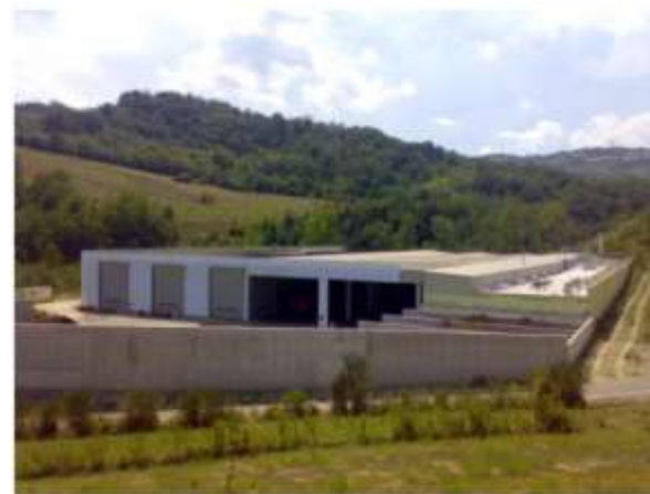
Centralized industrial plants
